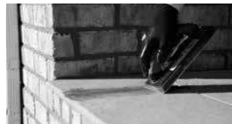
PIC 1. Fill joint with grout.
