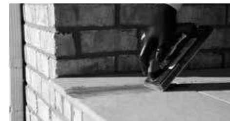
PIC 2. Remove excess grout with clean water.
